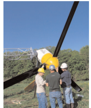
Bergey WindPower 10kW XLS turbine lowered for ground maintenance
