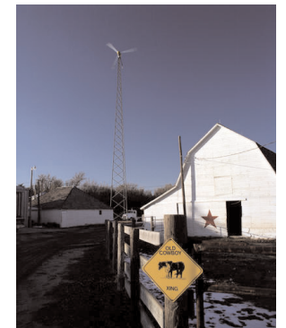
Bergey WindPower 10kW XLS turbine
