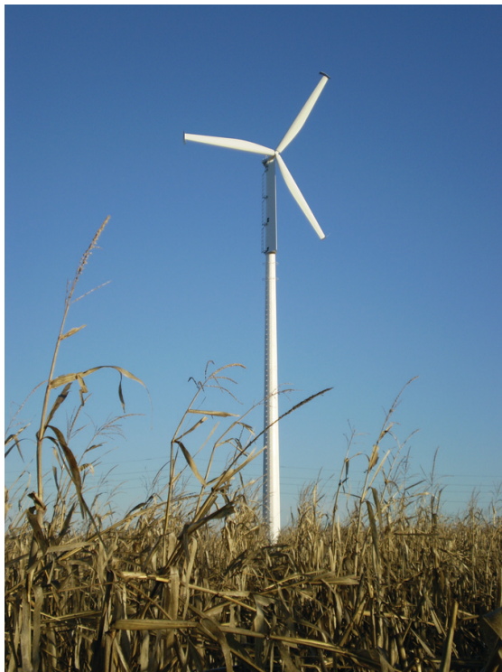
Entegrity Wind Systems 50kW turbine
