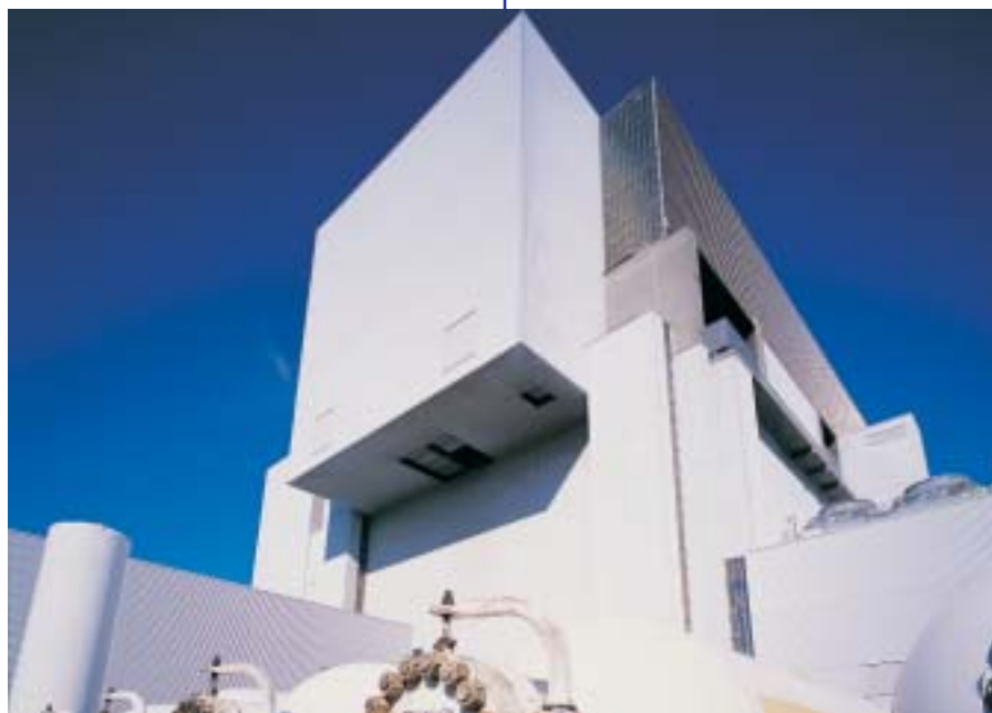
British Energy's Torness Power Station
