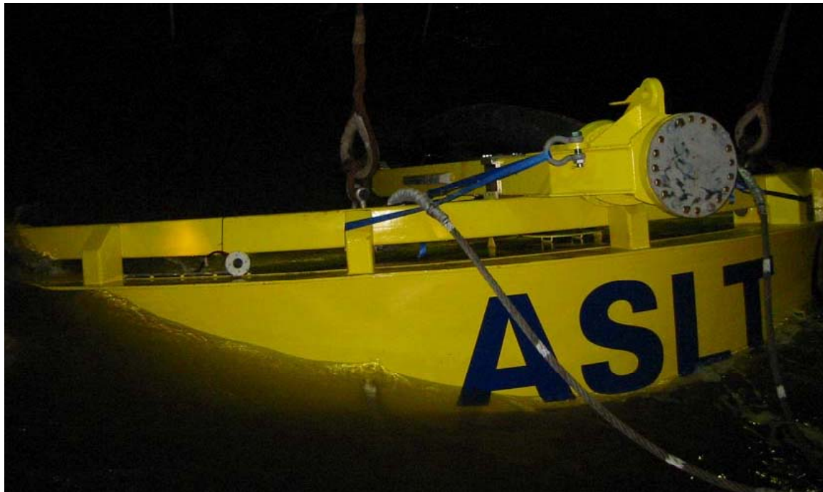
PLEM – as last seen prior to be submerged and installed at the place
