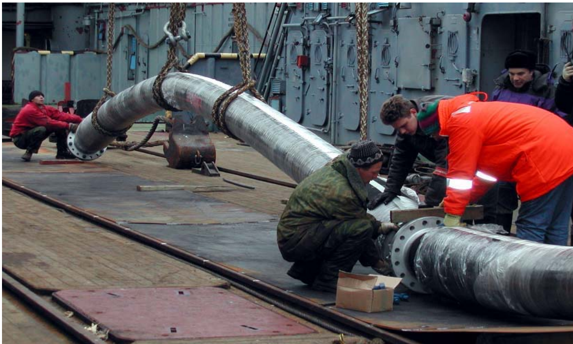
On-deck assembling of flexible connection between existing pipeline and PLEM
