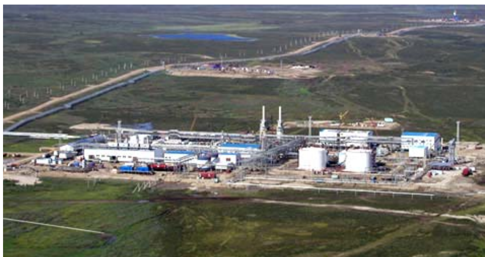
Central oil collecting point of SeverTEK at the Yuzhno-Shapkino field in Nenets AO
