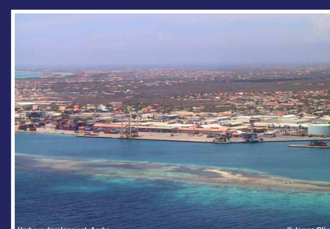
Harbour development, Aruba.
