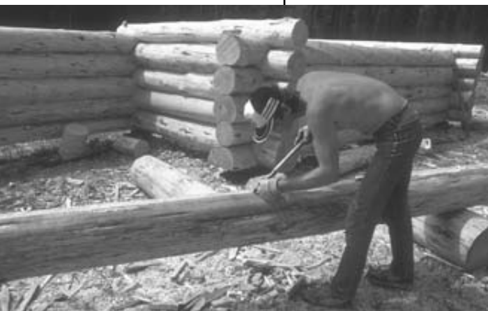
Building a log cabin, Yukon Territory.
