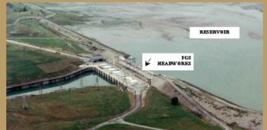
Pump Generating Station
