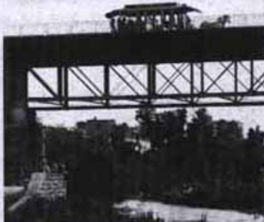
The Metropolitan Railroad's horse-drawn trolley crossing Rock Creek on P Street, leaving Dupont Circle for Georgetown. Courtesy LeRoy O. King, Jr. Photo by Handy Studios (1880's).
