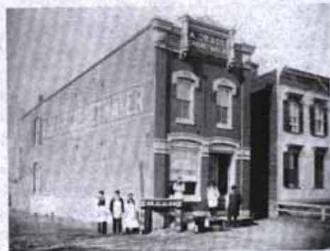
A. Grass cabinetmaker, 1209 New Hampshire Avenue. Demolished. Courtesy Historical Society of Washington, D.C.
