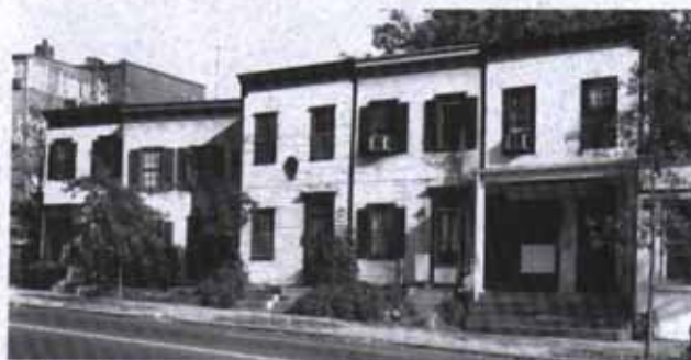
2120-2128 Florida Avenue (ca. 1868). Courtesy Kiplinger Washington Collection, W. E. Barrett photograph (1967).
