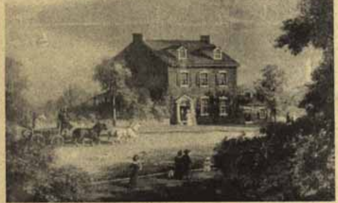
The home of Francis Scott Key, Georgetown attorney, educator, and author of The Star-Spangled Banner. Built 1802 and purchased by Key in 1805. The Georgetown-Leesburg Turnpike Road (M Street) in foreground. Demolished 1947 for construction of Whitehurst Freeway. The Francis Scott Key Park now marks the site at 34th and M Streets. Painted by John Ross Key, grandson of Key in the mid-1850s. Courtesy Peabody Room, Georgetown Public Library.
