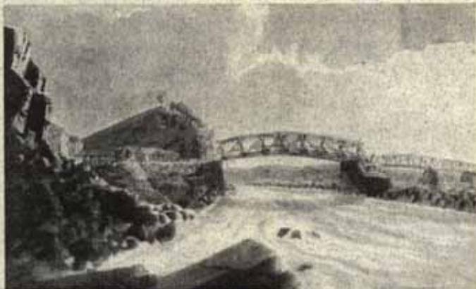
"Sketch of the Bridge at the little Falls of the Potowmack", by architect Benjamin Henry Latrobe, 1798. One of the earliest long trussed arch-bed bridges designed by Timothy Palmer. Technology first used in 1792. Pre-fabricated and shipped from Newburyport, Connecticut. Courtesy Maryland Historical Society.
