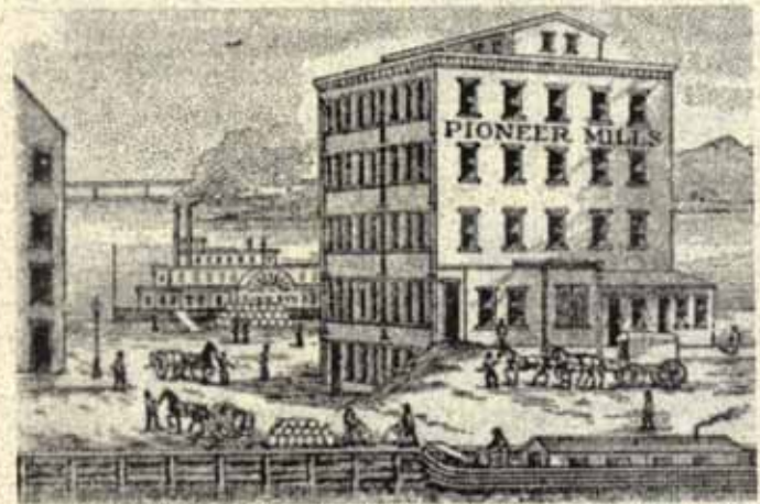
The Bomford Mill, 3261 K Street (1845-47). Built on site of 1832 flour mill, burned in 1844. Utilized water power from canal. Cotton mill 1847 to Civil War. Converted again to flour mill 1883. Note steamboat on river, canal with boat unloading in foreground. Boyd's Washington Directory, 1886.
