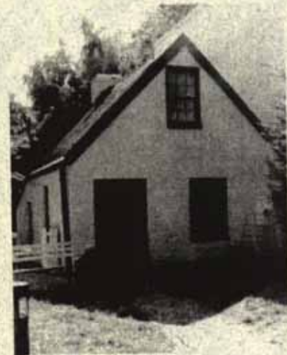
Community House of the Mt. Zion Church, 2906 O Street (1813). Residence of free black members of congregation. Surviving example of English cottage architecture. Restored as archives of African American life in Georgetown, with assistance of 1985 DCSHPO/HPF grant. Courtesy Mt. Zion United Methodist Church Archives.
