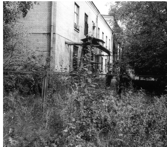
This building at the Kurchatov Institute in Moscow, shown before cooperative security upgrades began, holds enough HEU for a nuclear bomb. The barely visible fence is almost entirely overgrown, and there are no sensors or detectors to alert security forces to an intrusion; nor was there any detector to detect authorized workers removing nuclear material. Source: DOE
