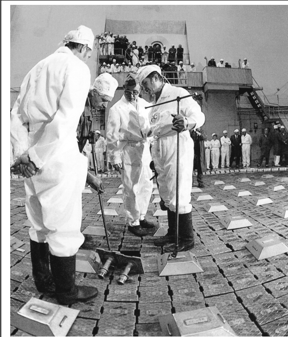
The top of the operating plutonium production reactor at Zheleznogorsk (formerly Krasnoyarsk-26), which produces half a tonne of weapons-grade plutonium each year. The United States and Russia are cooperating to convert this reactor and two more like it at Seversk (Tomsk-7) to a new fuel cycle that no longer produces weapons-grade plutonium, but the program is bedeviled by delays, cost-overruns, safety concerns, and nonproliferation issues related to the planned use of HEU fuel. Source: PNNL
