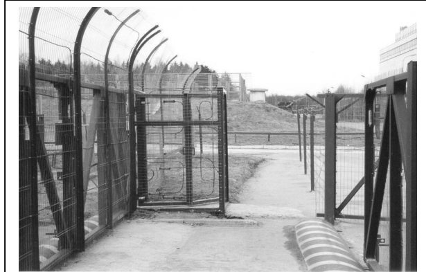
Fifty sets of security fencing such as that shown above are being provided by the Cooperative Threat Reduction program to help upgrade security at Russian nuclear warhead storage sites. Nuclear warheads are believed to be much more secure than fissile material, but even in this sector, low and intermittent pay and increasing reports of crime and poor morale have raised security concerns. Source: DOD
