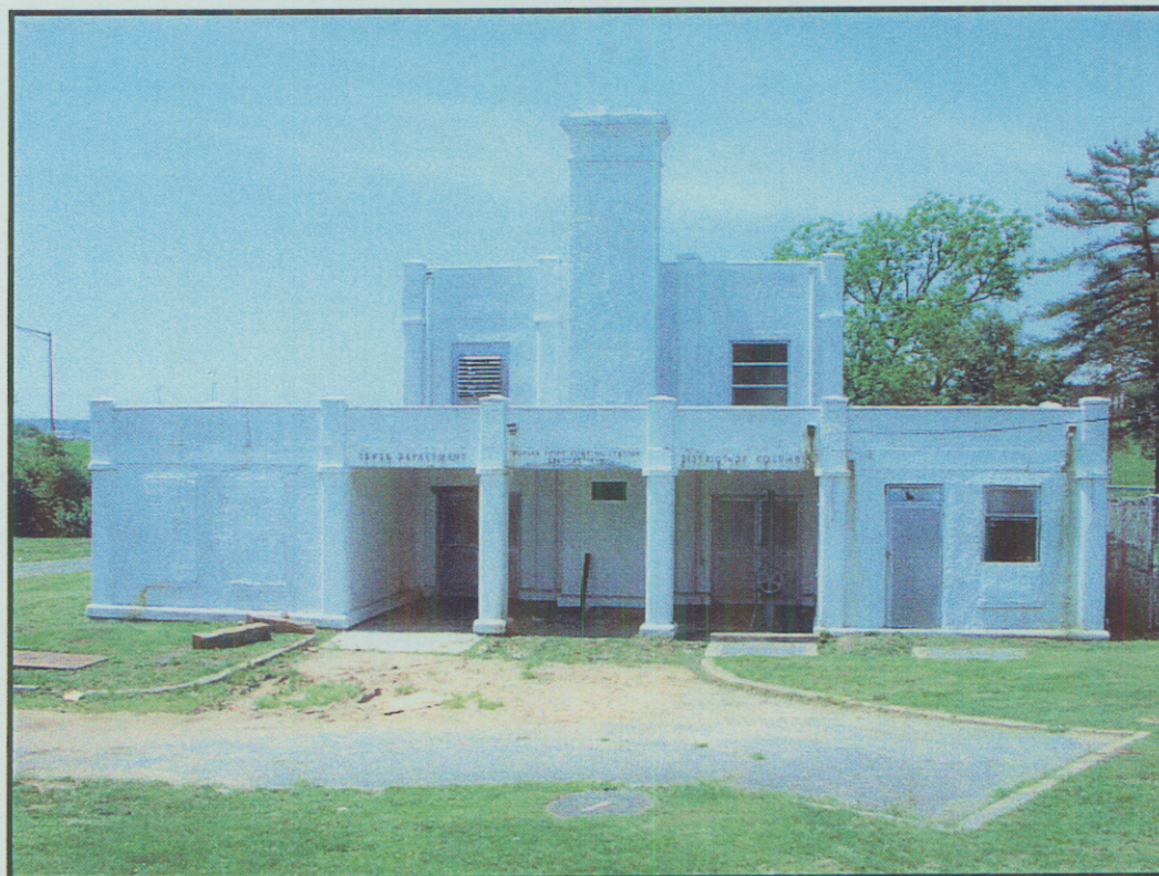
Photo 10: District of Columbia Poplar Point Sewage Pumping Station, facing west.
