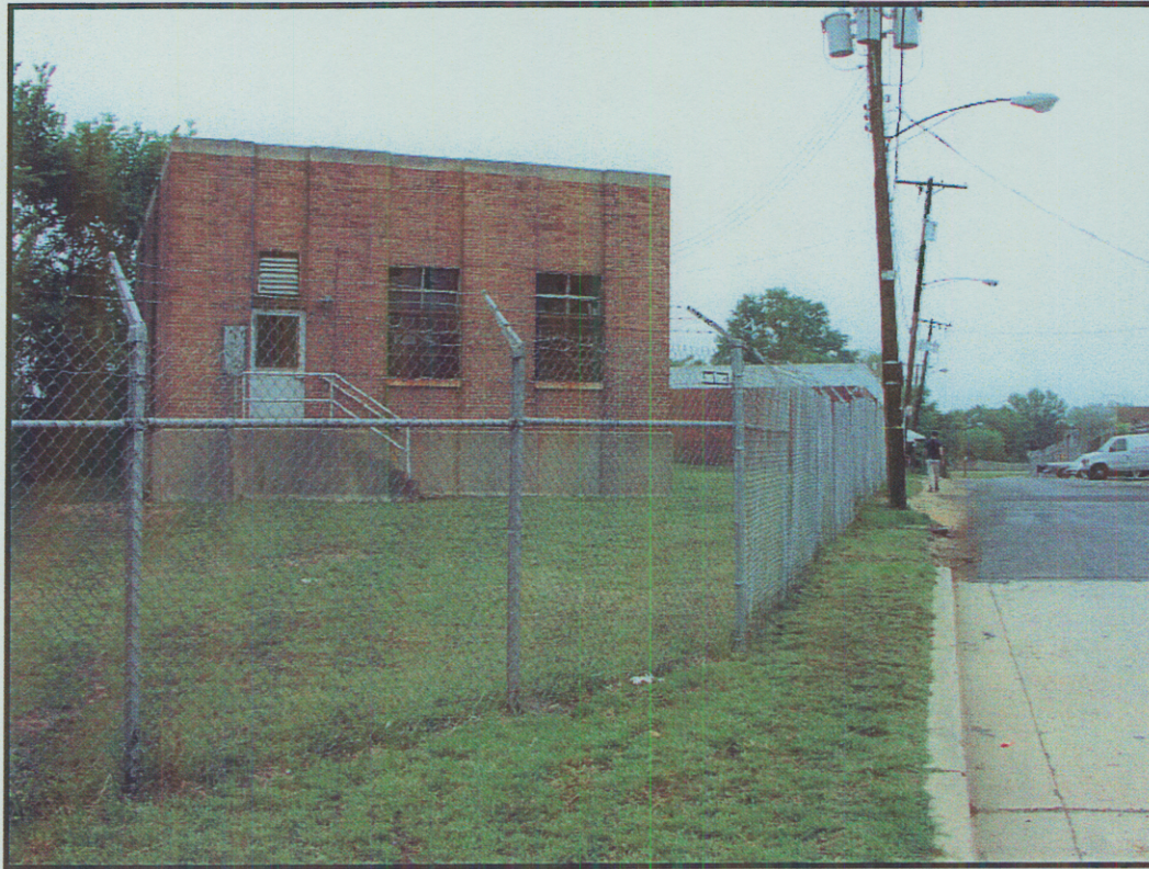
Photo 5: Overview of 5864-808, facing northeast. Note: pole mounted transformers on top right portion of photograph.
