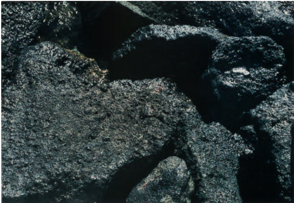
Figure 21B. Plot for high-pressure, hot-water washing alone on rip rap. Pressure and temperature were incrementally increased to 1,200 psi and 175°F. Smooth rock surfaces were cleaned much better than the rough surfaces.
