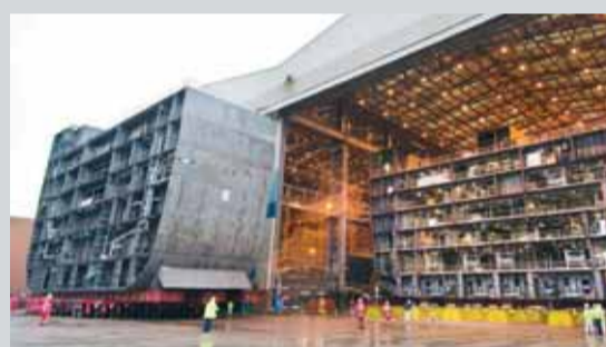
Above: the section beginning its 100 metre move across the shipyard
